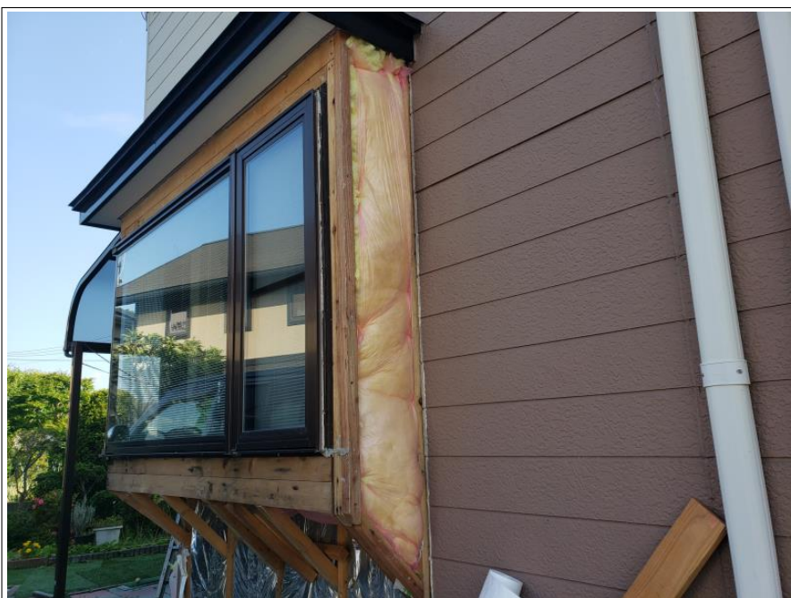
1階出窓部外壁
