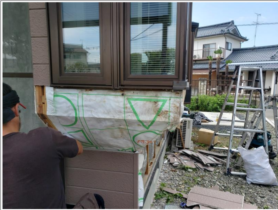
1階出窓部外壁
