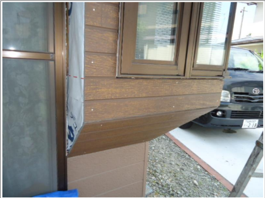
1階出窓部外壁
