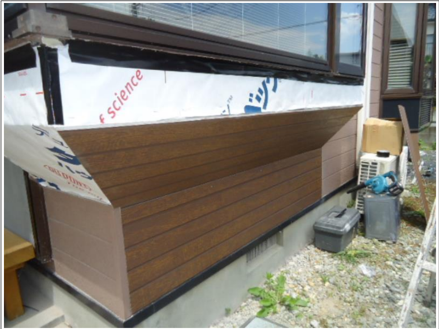
1階出窓部外壁
