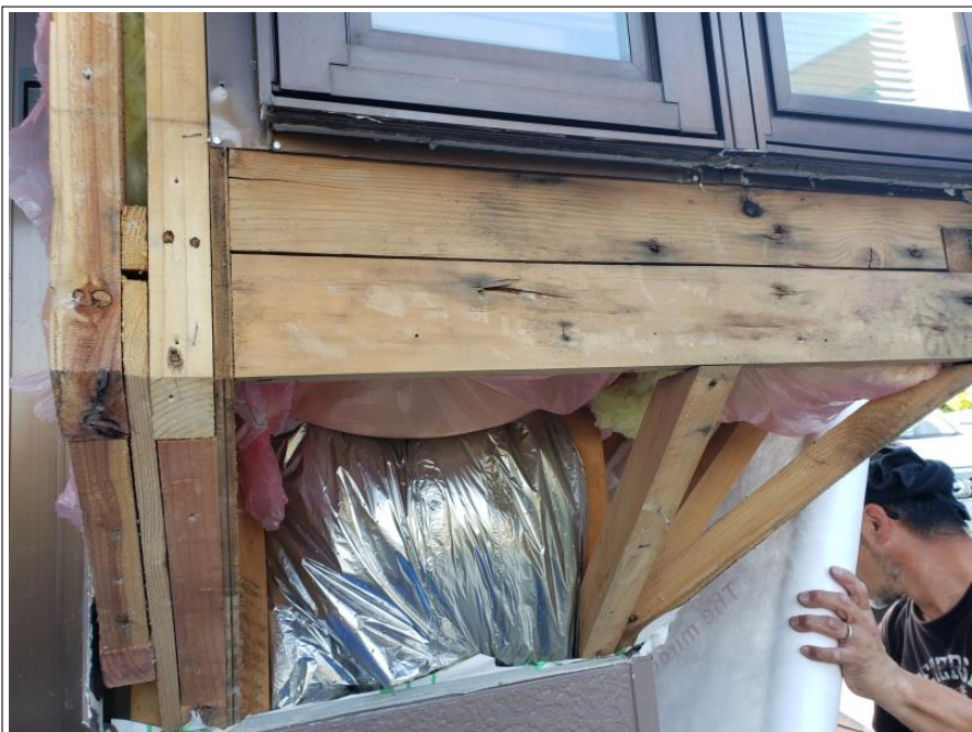
1階出窓部外壁
