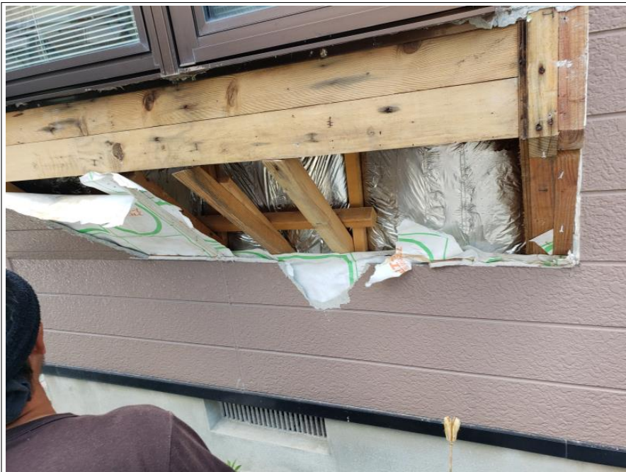
1階出窓部外壁
