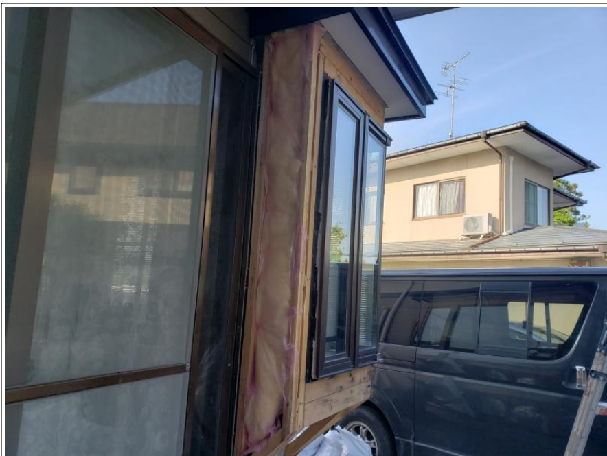
1階出窓部外壁
