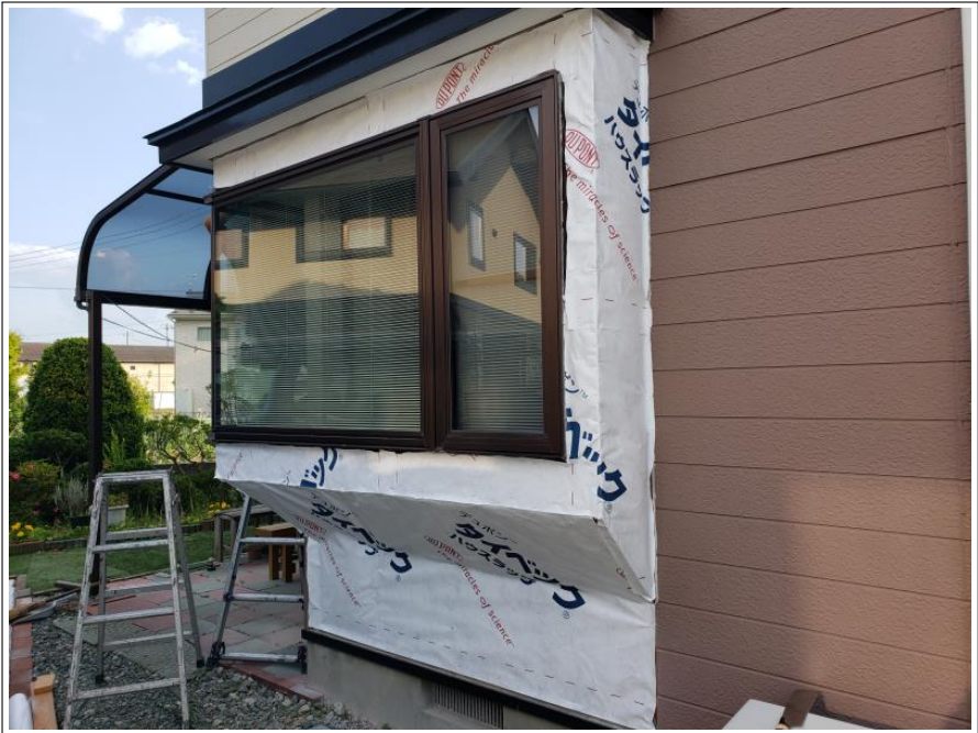
1階出窓部外壁
