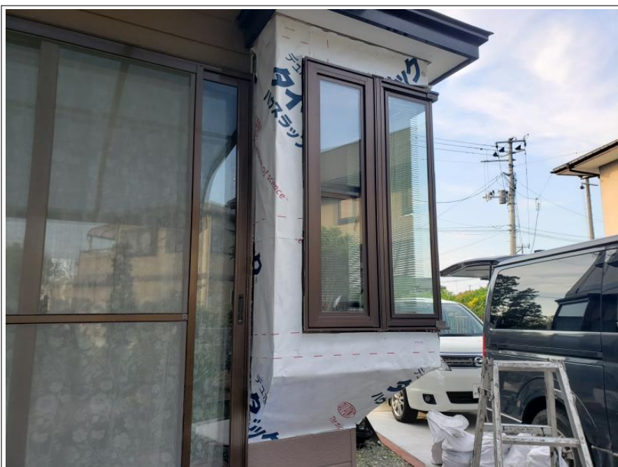
1階出窓部外壁
